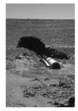
A) Avoid placing the conduit across compressible soil zones or close to filters.
